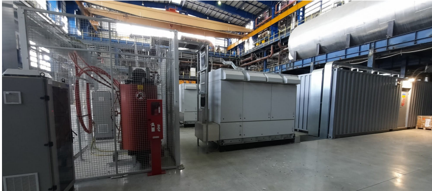
Figure 35: Photo of the transformer, PCS group and battery subsystem from the side
