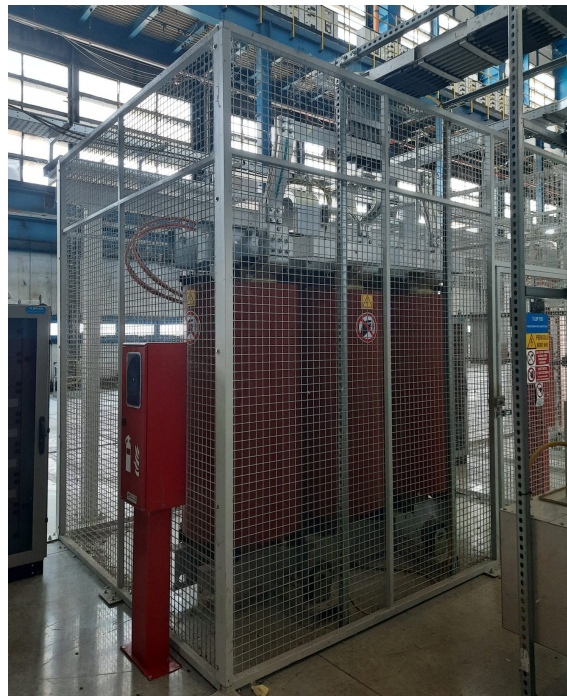
Figure 38: Detail of the Turbigo Tranformer
